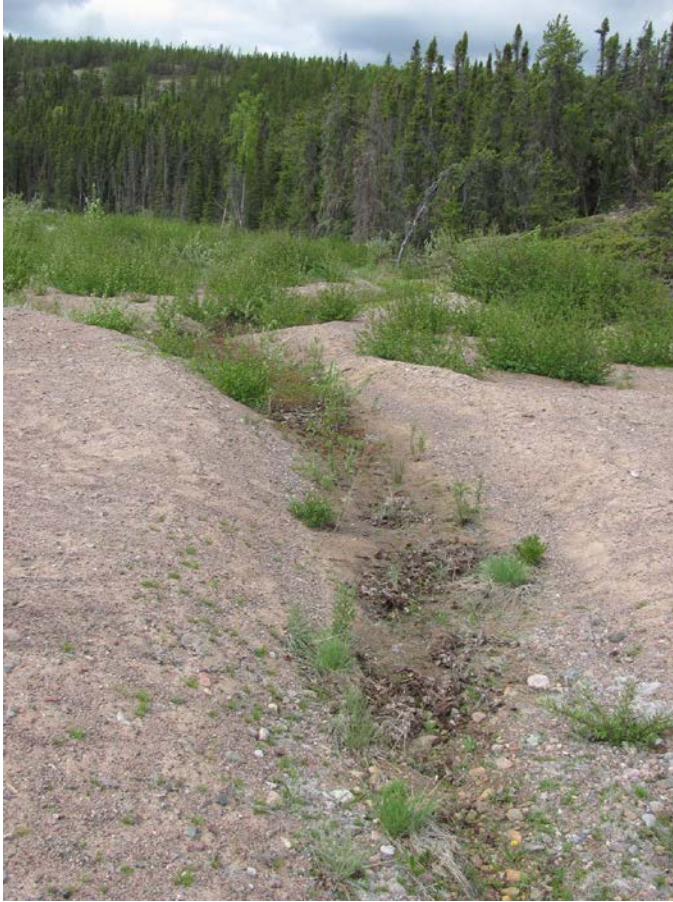
Photo 9 – Vegetation growth near drainage trench on the Fookes delta
