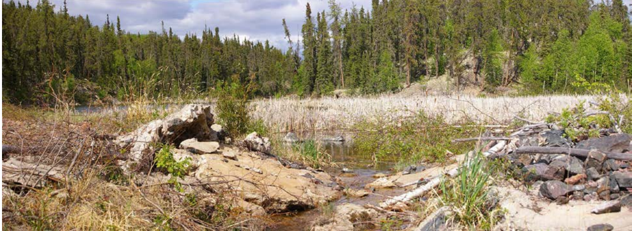
Photo 1 – Marie Reservoir Spillway looking upstream
