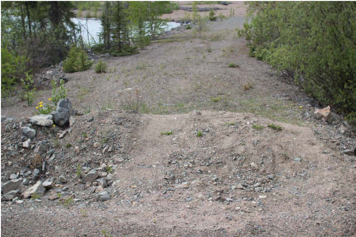
Photo 12 – East berm showing tire tracks driving over control point
