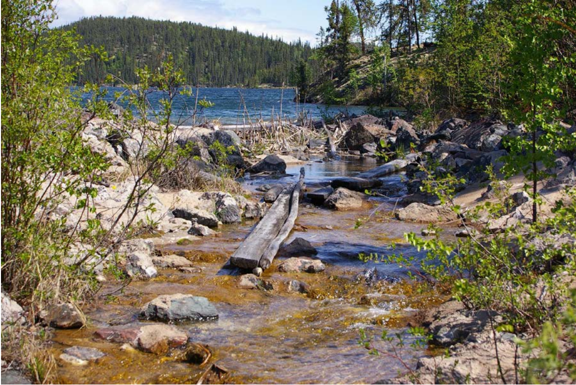
Photo 4 – Fookes Reservoir Spillway looking upstream
