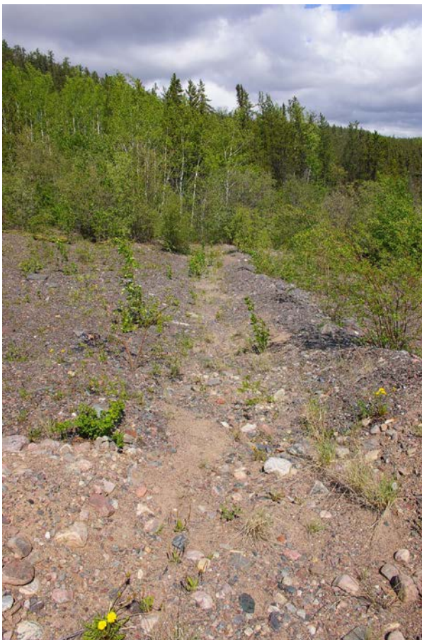
Photo 11 – Run-out structure along north access road
